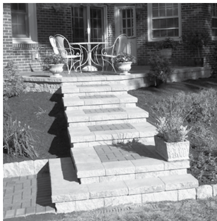
Figure 4-21: Straight parallel outset steps.
