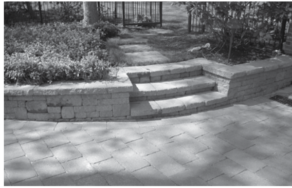
Figure 4-23: Outside curve parallel inset steps.
