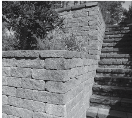
Figure 4-14: Steps constructed with SRW units.
