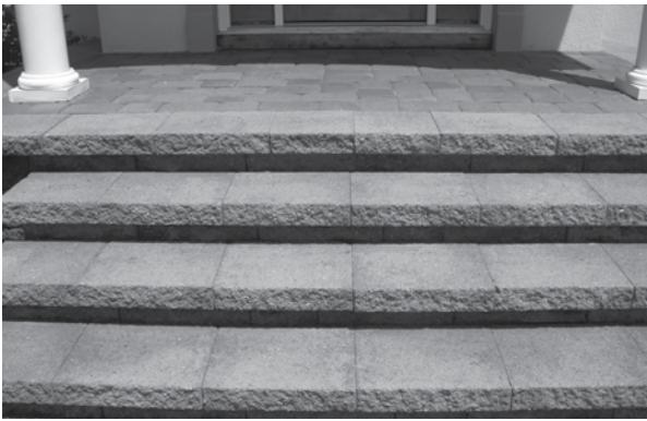
Figure 4-24: Straight parallel outset steps.
