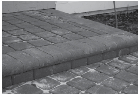
Figure 4-18: Bullnose pavers used for treads.
