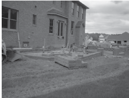
Figure 4-33: Staging materials and equipment will help keep a work site productive
