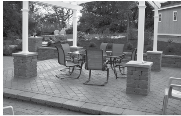
Figure 4-25: A raised patio with only one riser.
