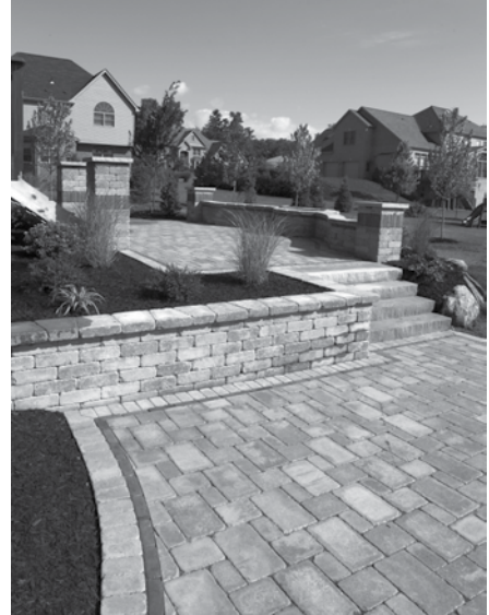
Figure 4-2: This raised patio used a seat wall as a guard. This is not acceptable according to some building codes.
