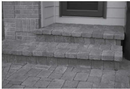
Figure 4-17: Steps constructed using pavers.
