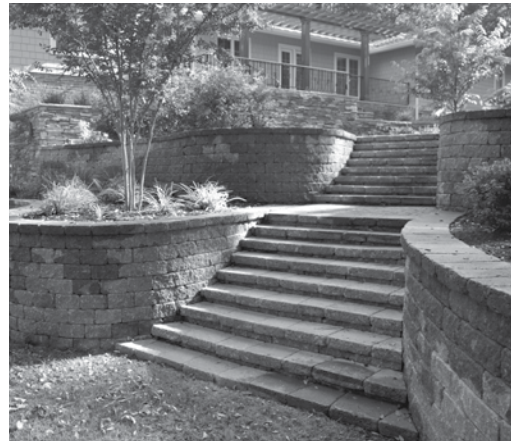
Figure 4-20: Double set of parallel inset steps.
