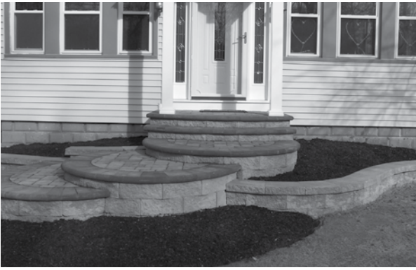
Figure 4-22: Round outset steps using bullnose treads.
