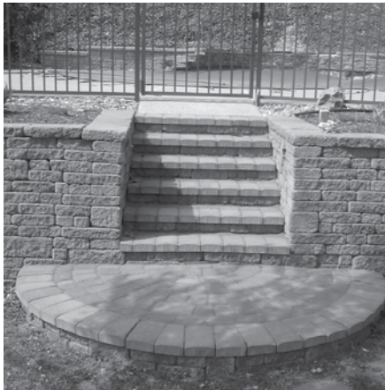
Figure 4-19: Straight parallel inset steps using pavers as treads with a lower outside curved landing.
