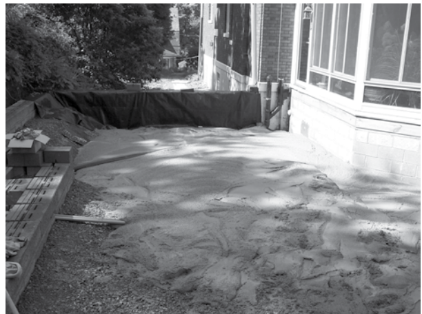
Figure 4-35: Even though flowable fill may be more expensive than aggregate, it may require less labor on some projects.
