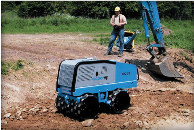
Figure 2. Compacting the soil subgrade.
