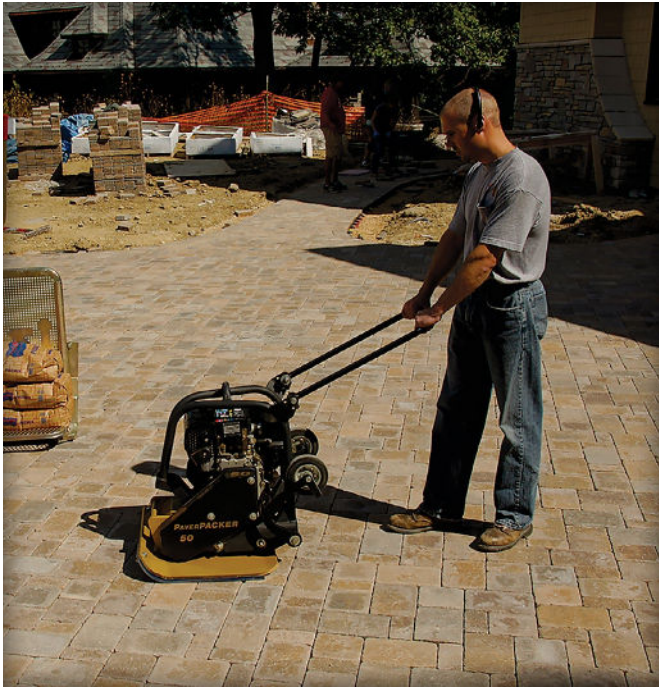
Figure 9. Compacting the pavers and bedding sand.
