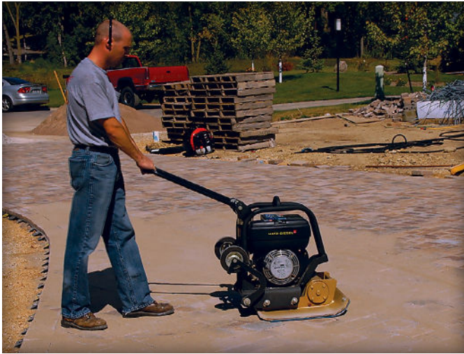
Figure 11. Vibrating sand into the joints.
