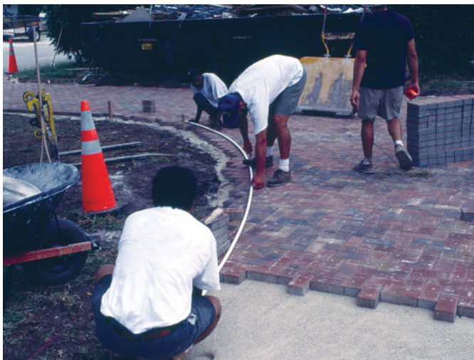
Figure 13. Marking pavers for saw cutting. The cut pavers are carefully removed and edging is placed against the pavers.
