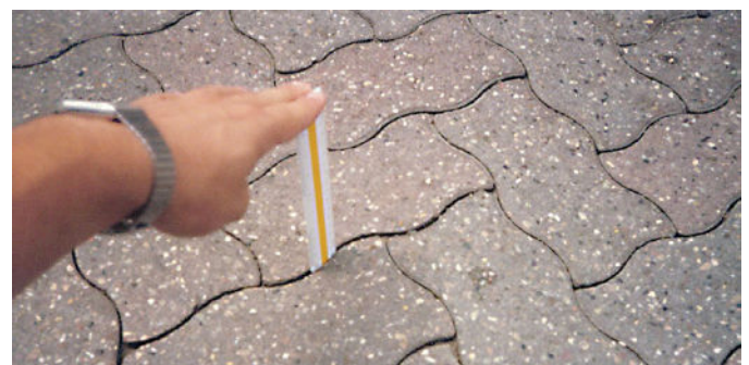
Figure 2. Refill joints with dry masonry sand if loss is greater than 1/2 in. (12 mm).
