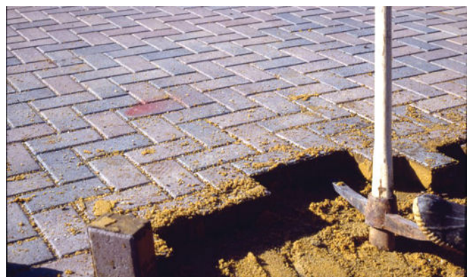
Figure 32. A pick or pry bar can be used to reach under the pavement edge and pry units out.
