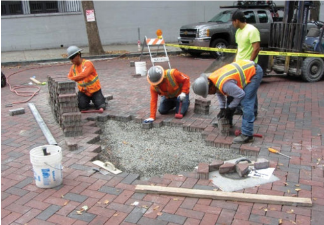
Figure 40. Pavers salvaged during the disassembly can be brought back and placed according to the original pattern. Care needs to be taken to ensure any remaining sand on the bottom or sides of the pavers is removed before placement.
