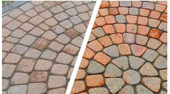
Figure 14. Cleaning the ICP surface can remove fine particles lodged in the pores of the concrete surface to rejuvenate the color.
