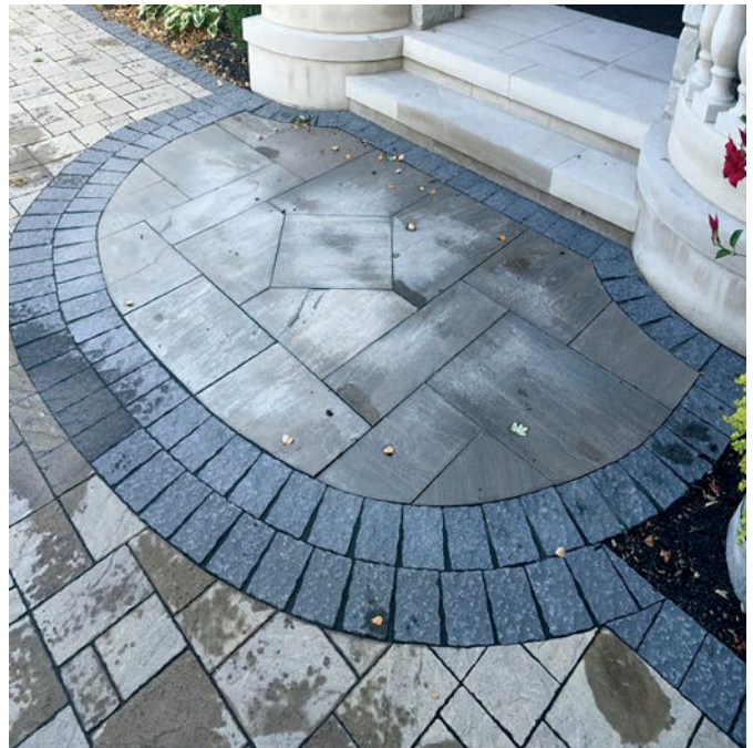
Figure 9. Efflorescence is only an aesthetic concern and can be removed with cleaners specifically formulated for this task.
