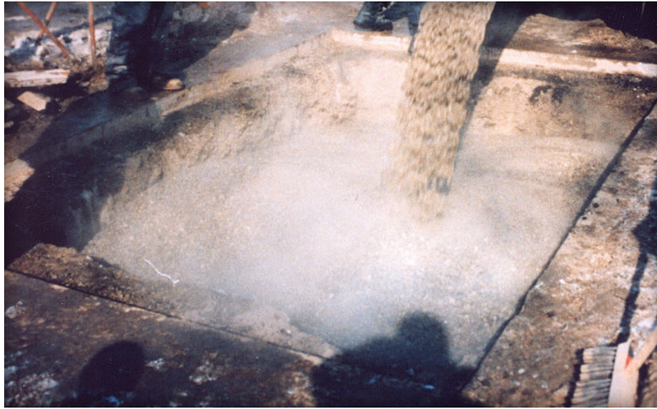
Figure 8. Low density concrete fill (unshrinkable fill) poured into a utility trench from a ready-mix concrete truck.
