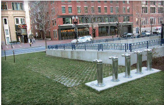
Figure 7. Emergency access lane for fire trucks
