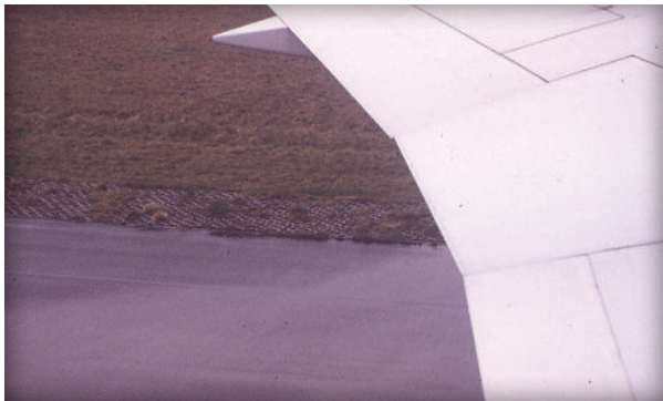
Figure 11. Airfield taxiway shoulder
