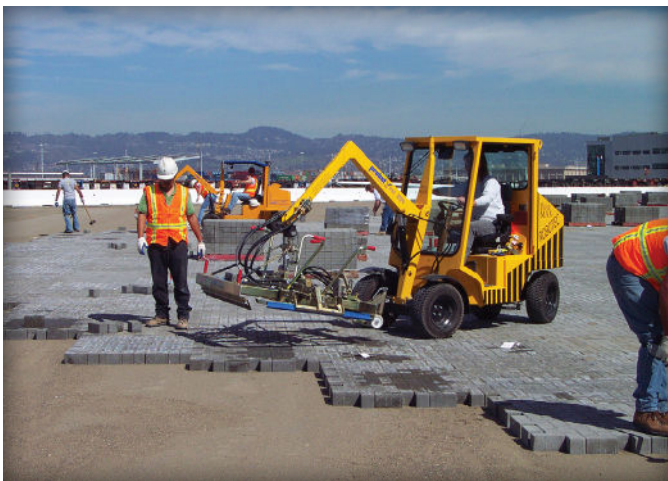
Figure 5. Motorized equipment with a hydraulic clamp.
