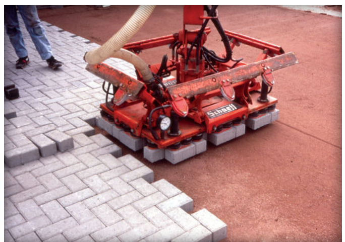
Figure 6. The vacuum head over the paver layer.
