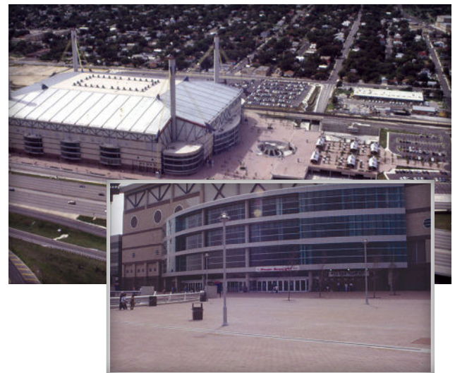
Figure 22. The plaza area around Scope Center in Norfolk, Virginia, (left) and one side of the Alamo Dome (right) in San Antonio, Texas, include roof plaza decks surfaced with concrete pavers.
