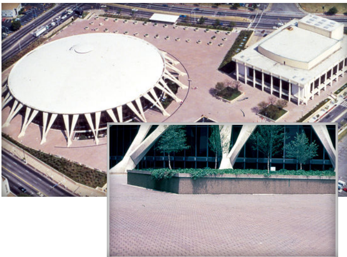
Figure 22. The plaza area around Scope Center in Norfolk, Virginia, (left) and one side of the Alamo Dome (right) in San Antonio, Texas, include roof plaza decks surfaced with concrete pavers.
