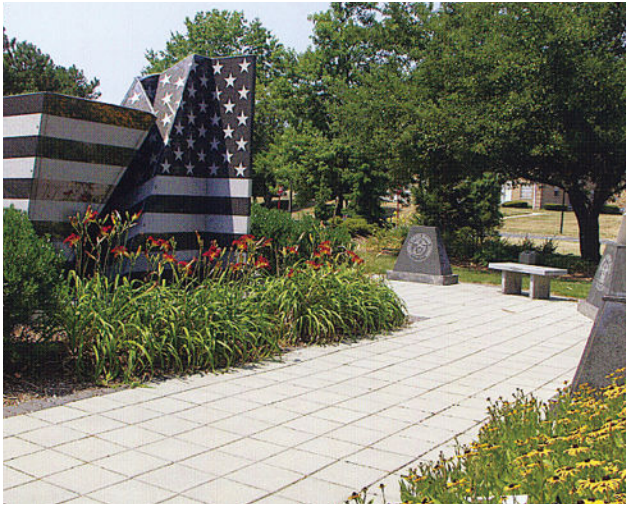
Figure 14. High SR paving slabs
