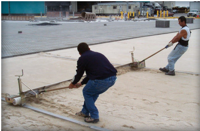
Figure 4. A two-man hand pulled screed
