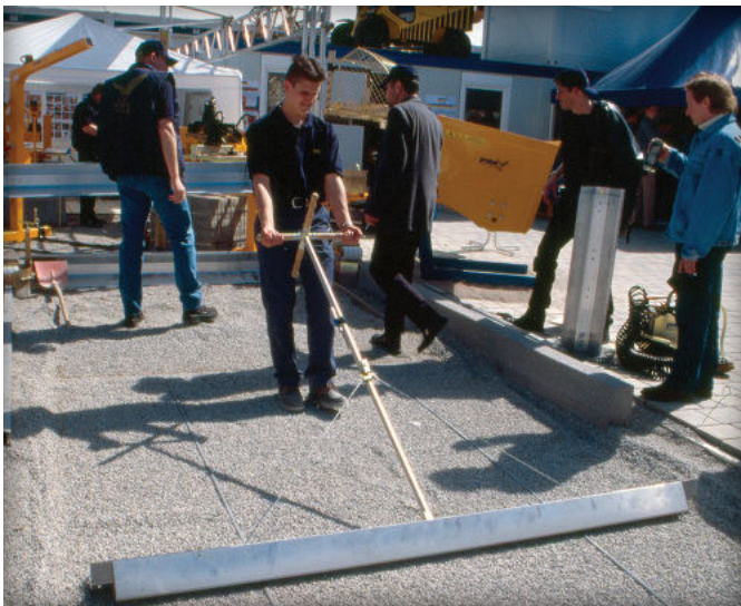
Figure 24. Manually screeding the No. 8 stone setting bed.
