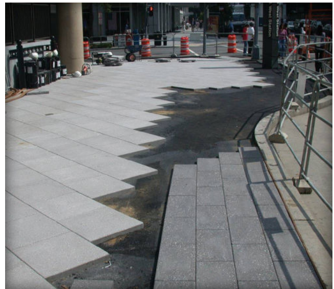
Figure 18. Paving slabs adhered to a bitumen-sand bedding in a Washington, DC, sidewalk.
