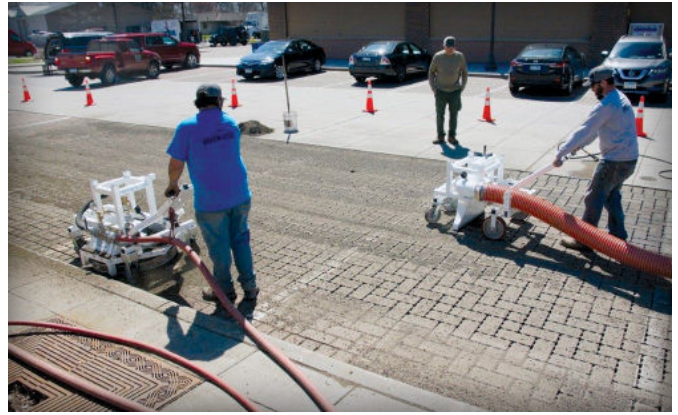
Figure 24. This equipment blows sediment and soiled aggregate from the joints and uses vacuum equipment to remove them.
