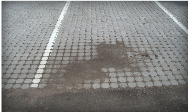
Figure 10. Erosion of adjacent asphalt and sediment deposition on PICP.
