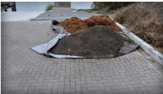
Figure 5. Mulch placed on tarps prevents more expensive cleaning of PICP.
