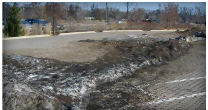
Figure 26. This is an example of snow that should have been deposited on a grassy area. If such areas are not available, then vacuum clean the PICP in the early spring.
