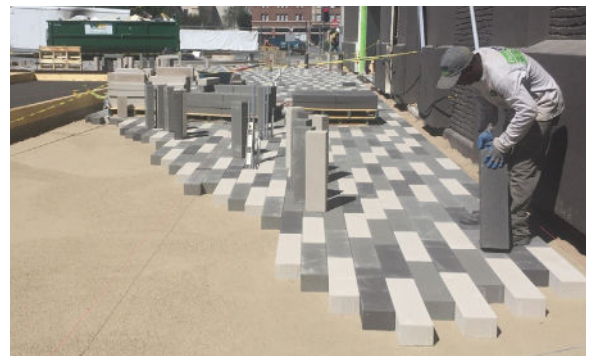
Figure 6. Installing planks on uncompacted bedding sand.
