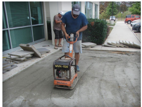
Figure 5. Precompacting the bedding sand
